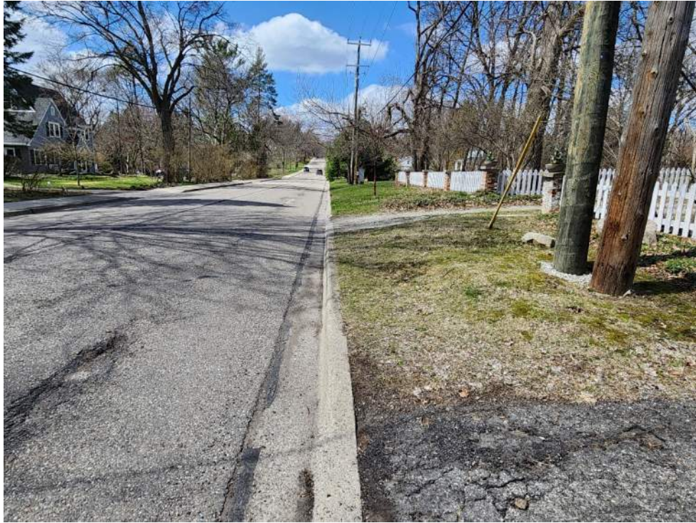
Sunset Road east of Foundation Drive looking west along the north side of the road
