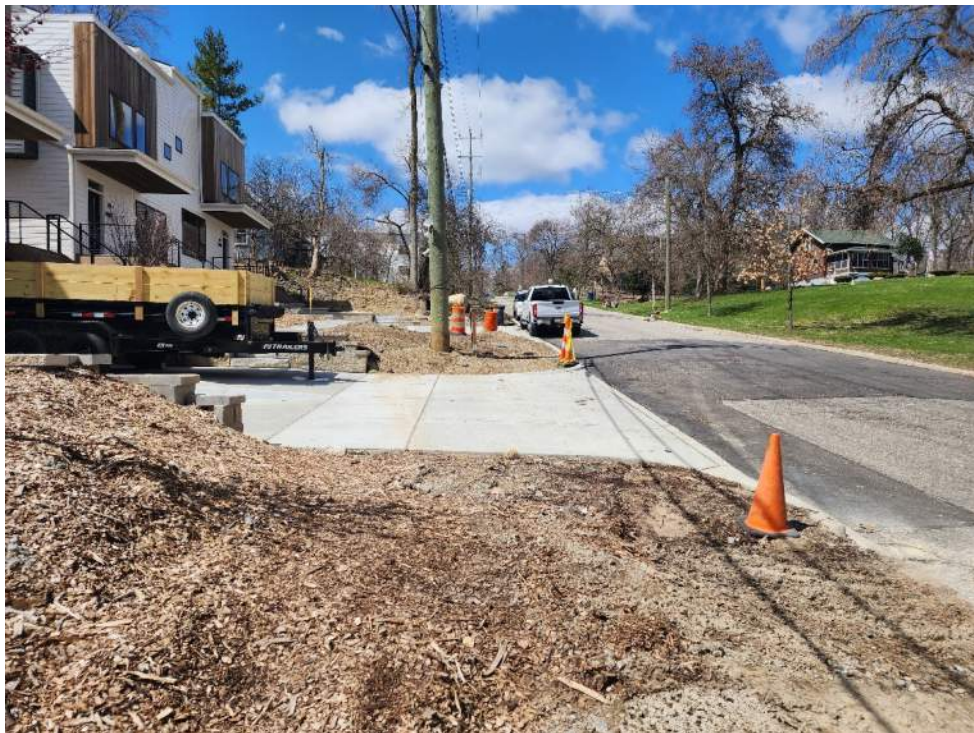
New condominium development north of Wildt Drive looking west along the south side of the road.
