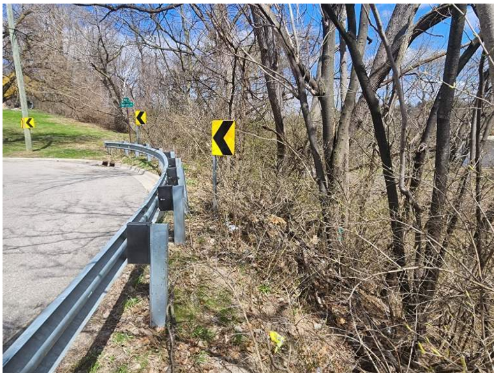
Outside portion of the 90° intersection of Sunset Road and Wildt Drive looking north from Wildt Drive. A significant drop off exists along the curve.
