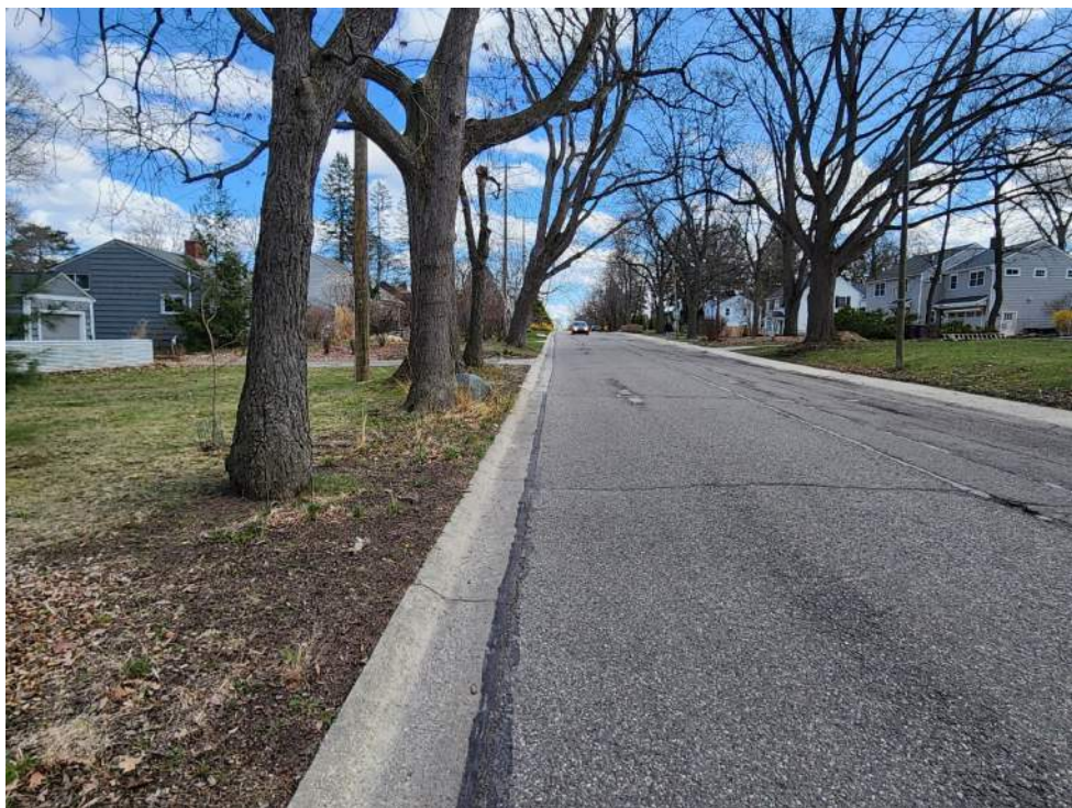
Sunset Road east of Brooks Street looking east along the north side of the road.
