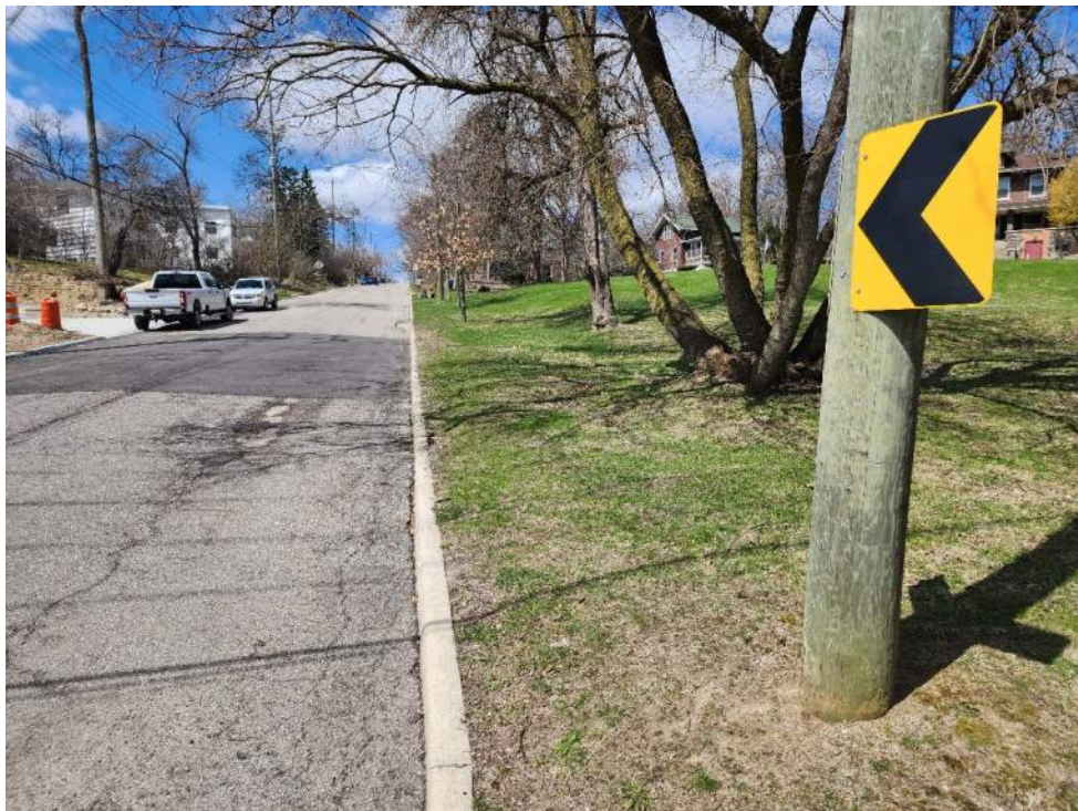
Sunset Road west of Wildt Drive looking west along the north side of the road.
