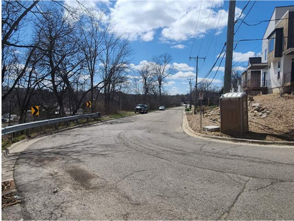
Intersection of Sunset Road and Wildt Drive looking south along the west side of the road.
