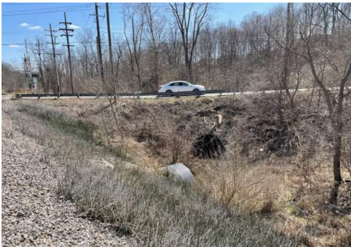
B1 Existing Condition: North side of Dhu Varren Rd, looking south
