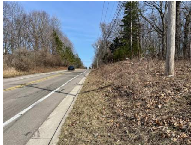
C2 Existing Condition: South side of Dhu Varren Rd, looking east
