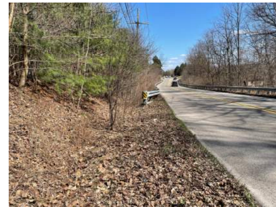
D1 Existing Condition: North side of Dhu Varren, looking east
