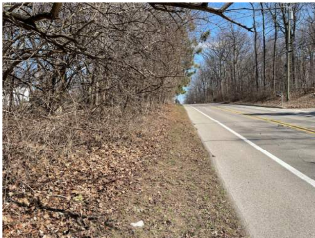
C1 Existing Condition: North side of Dhu Varren Rd, looking east
