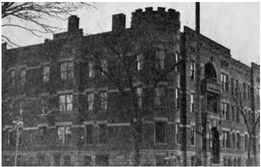
Left: Cutting Apartment Building - 1906
