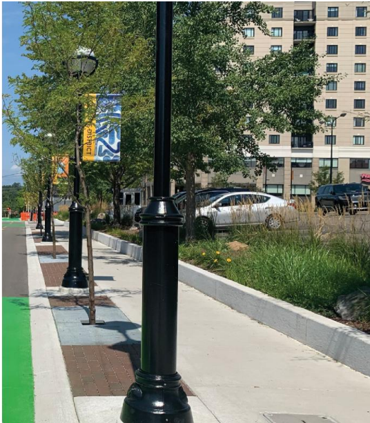
Brown and gray brick pavers
