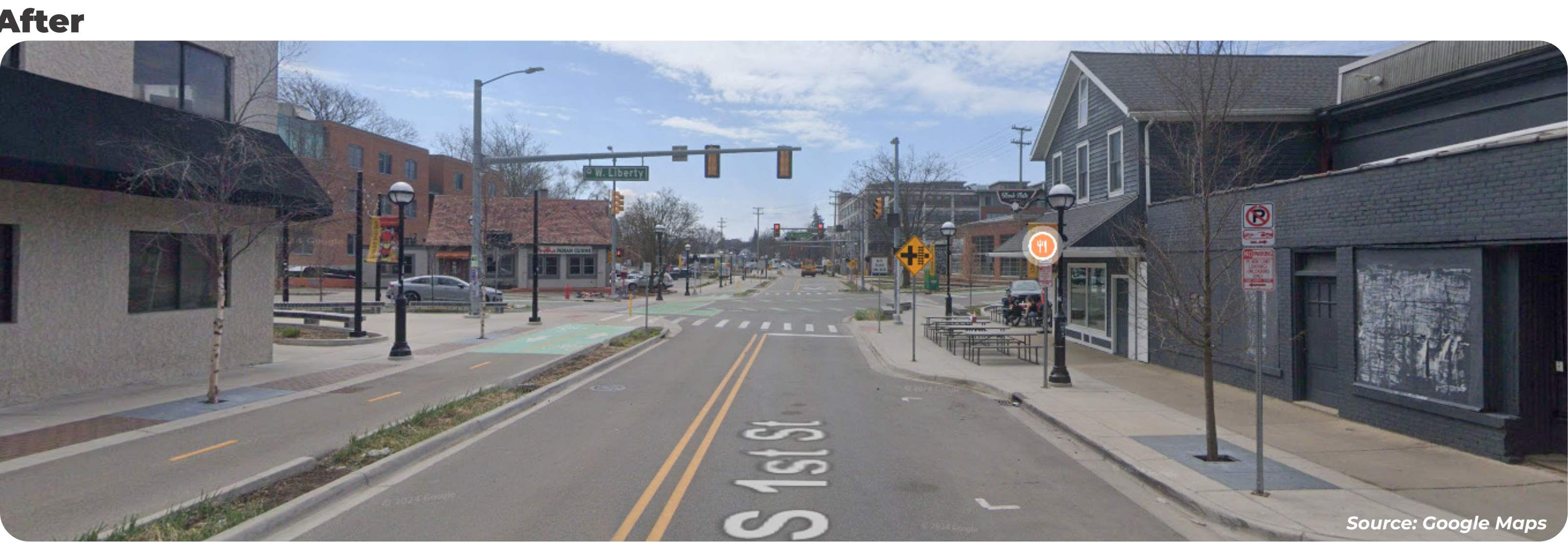
Image shows First Street and Liberty Street showing a separated bike lane with new curb extensions, roadway markings, and bike crossings.
