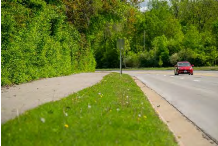
Curb and Gutter
