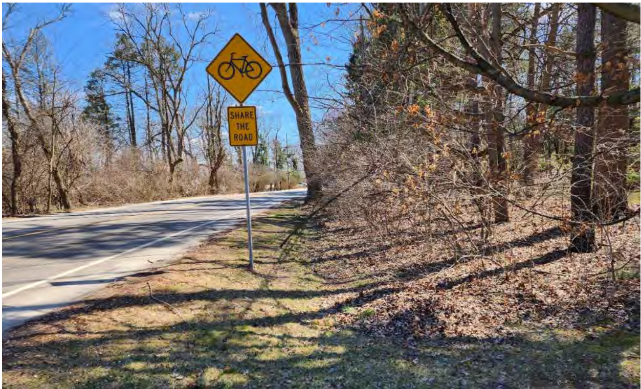
350 feet east of Blakeway looking east along the south side of Huron River Drive (preferred alignment)
