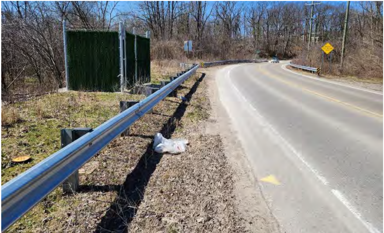
350 feet east of Chalmers looking west along the south side of Huron River Drive. A DTE Gas pressure reduction station lies inside the fence ( preferred alignment )
