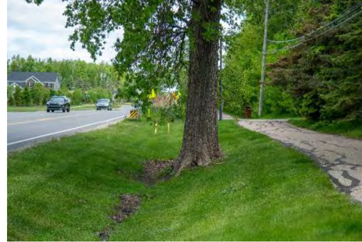
Shoulder with Ditch
