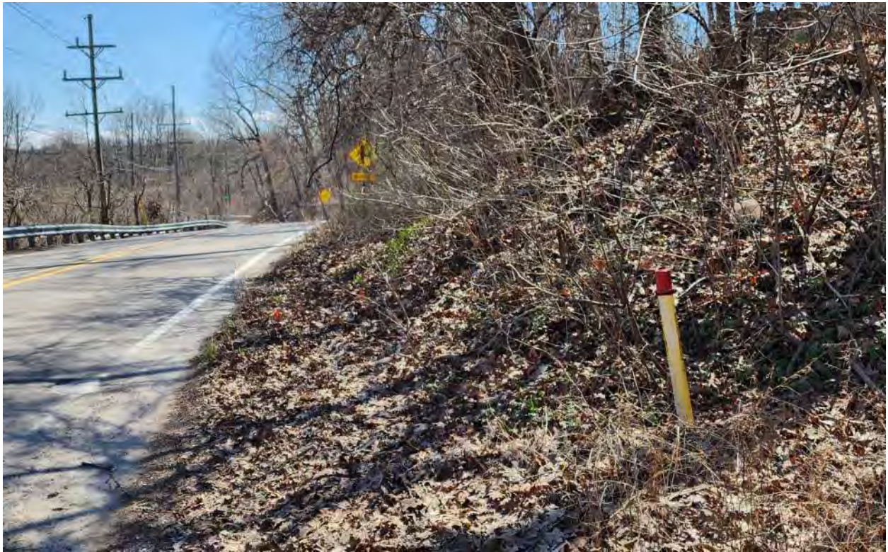
100 feet west of Chalmers Drive looking east along the south side of Huron River Drive (preferred alignment)
