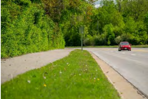
Curb and Gutter
