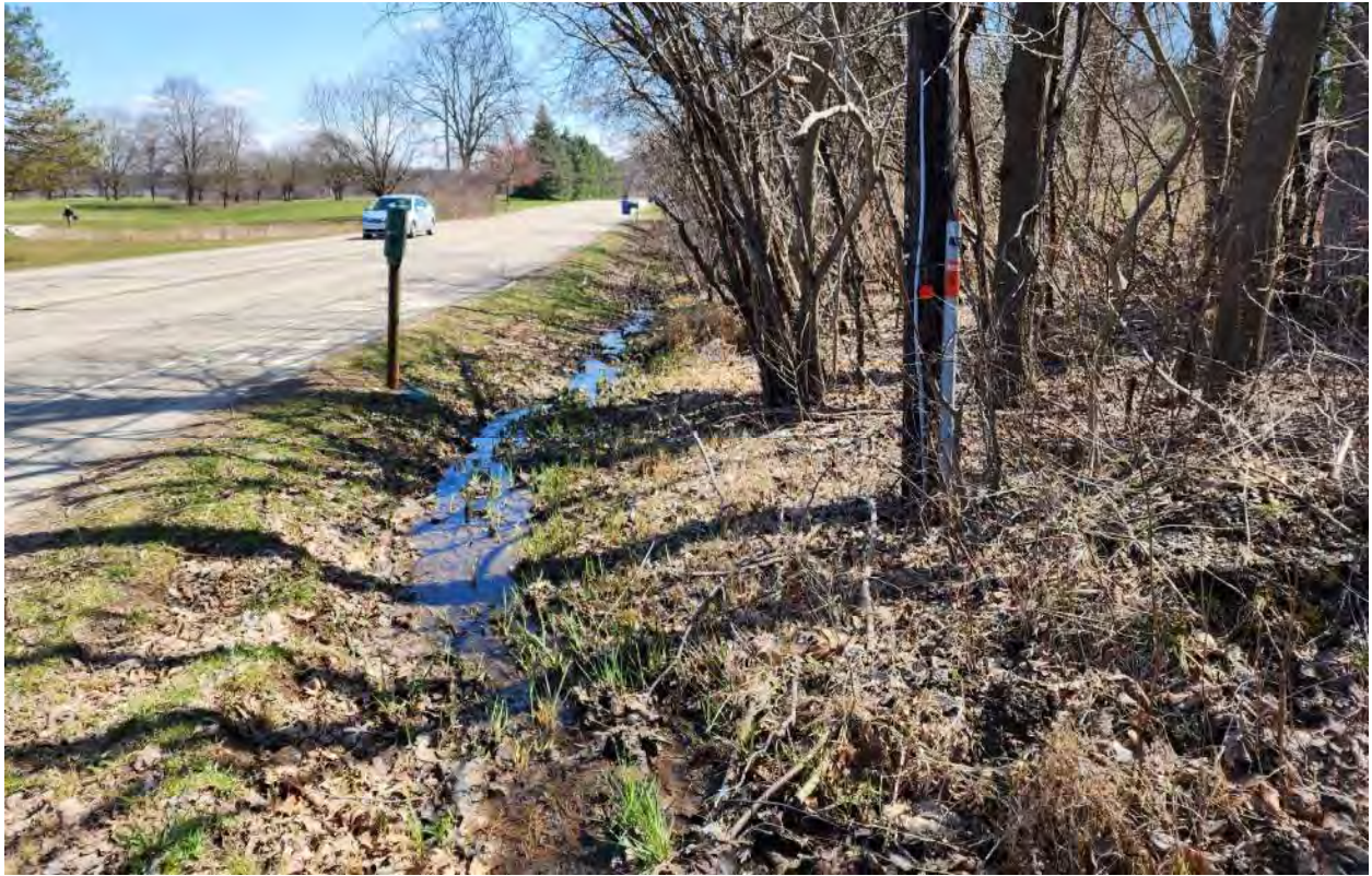
Southeast corner of Huron River Drive at Elmwood looking east
