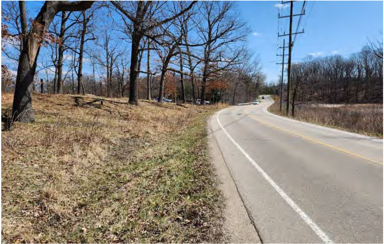
650 feet west of Thornoaks Drive looking east along the north side of Huron River Drive. (preferred alignment)
