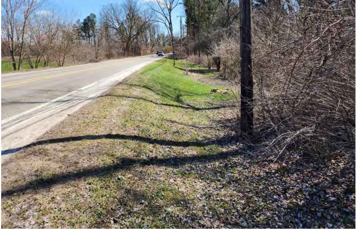
100 feet east of Blakeway looking east along the south side of Huron River Drive (preferred alignment)
