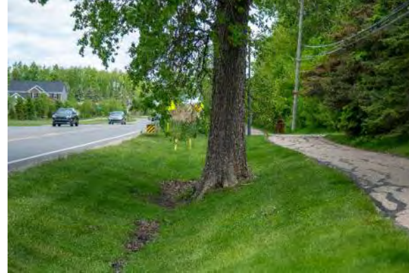
Shoulder with Ditch
