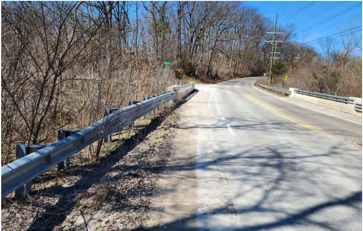
100 feet east of Chalmers looking west along the south side of Huron River Drive (preferred alignment)
