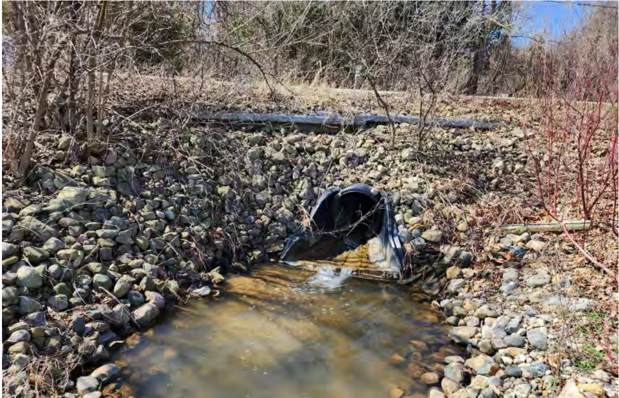
Outlet point into Benz County Drain
