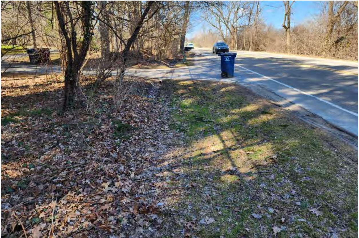
300 feet west of Woodland Drive looking east along the south side of Huron River Drive (preferred alignment)
