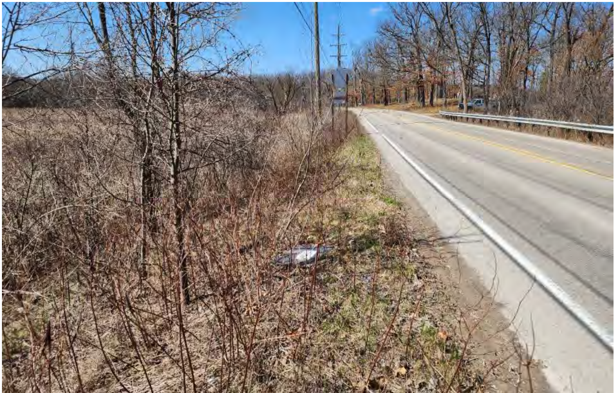
200 feet west of Thornoaks Drive looking west along the south side of Huron River Drive.
