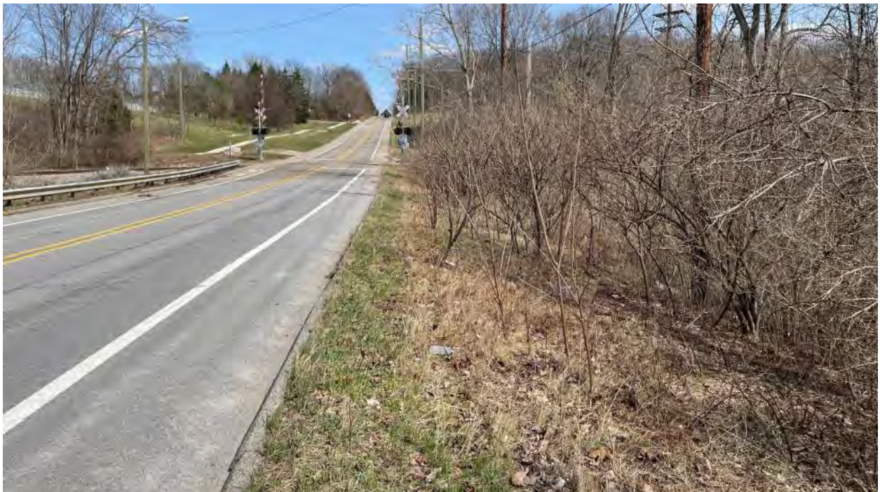
200 feet west of Ann Arbor Railroad looking east
