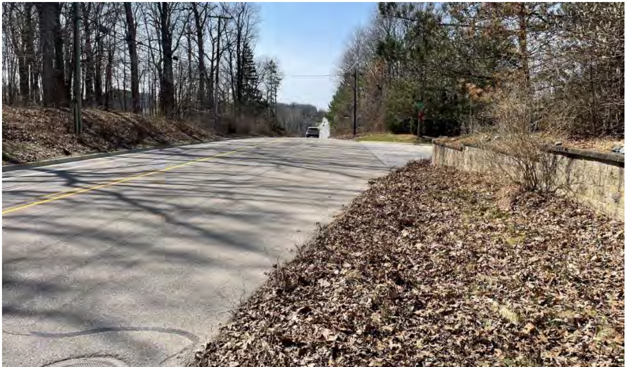
100 feet east of Birchwood Drive looking west
