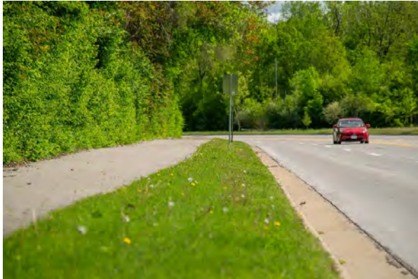
Curb and Gutter
