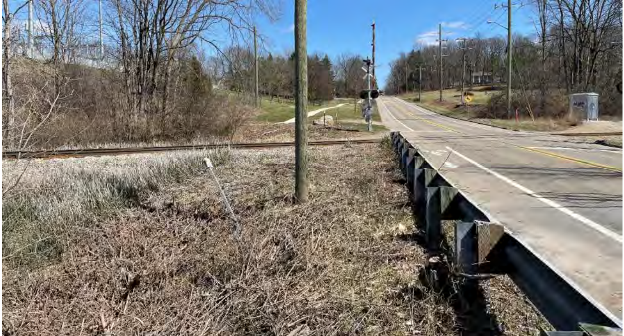
150 feet west of Ann Arbor Railroad looking east at the Traver Creek crossing.
