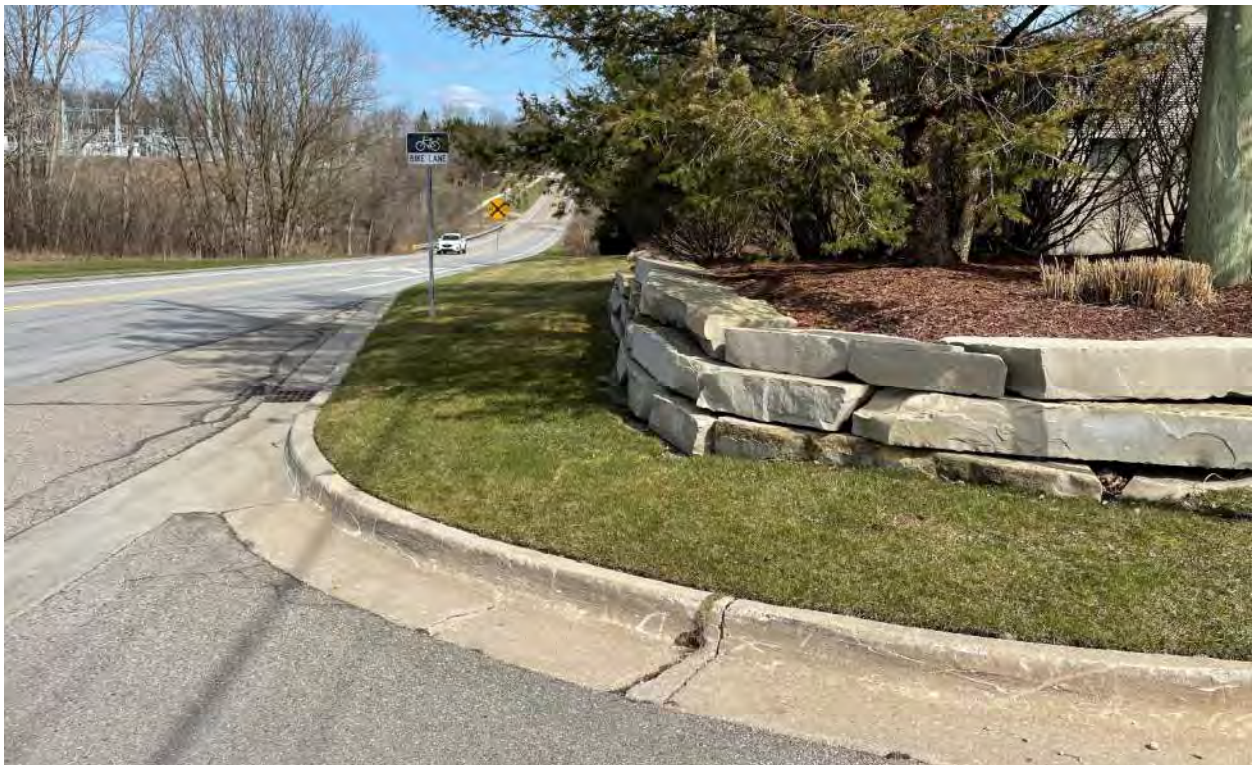
Intersection of Leslie Park Circle looking east
