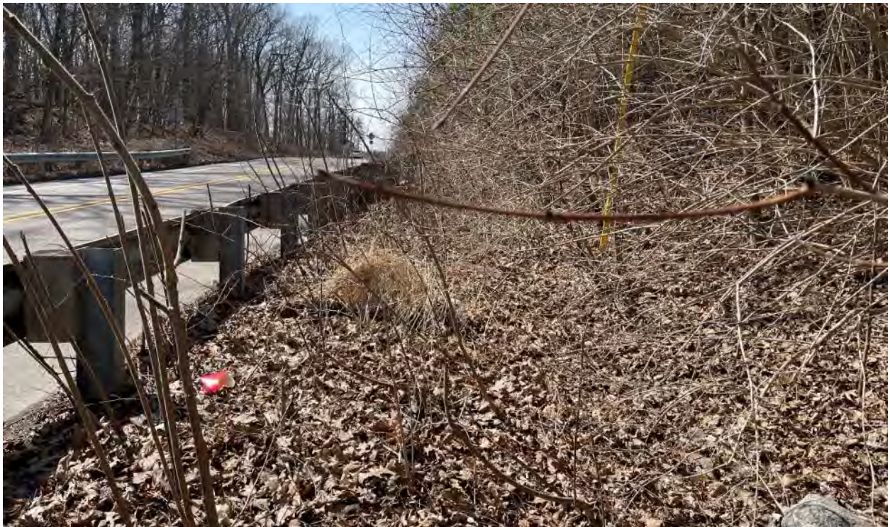
350 feet east of Birchwood Drive looking west
