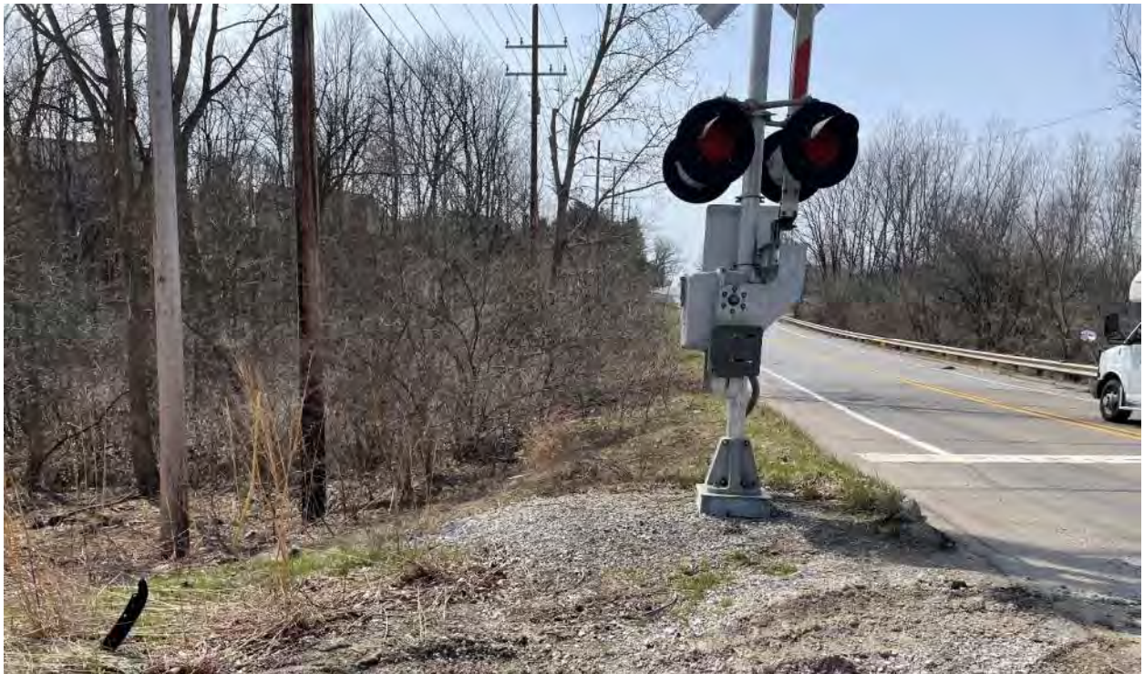
At Ann Arbor Railroad looking west
