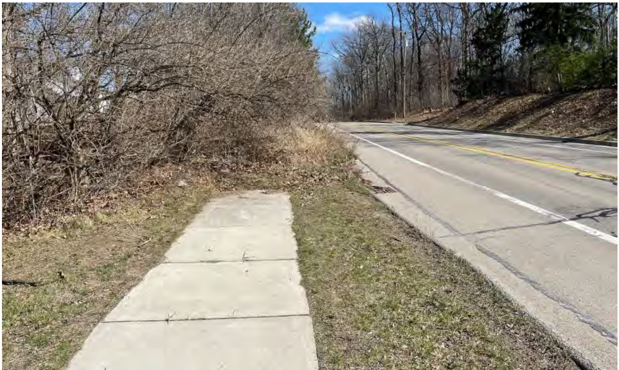
400 feet west of Birchwood Drive looking east. Sidewalk ends at DTE substation.
