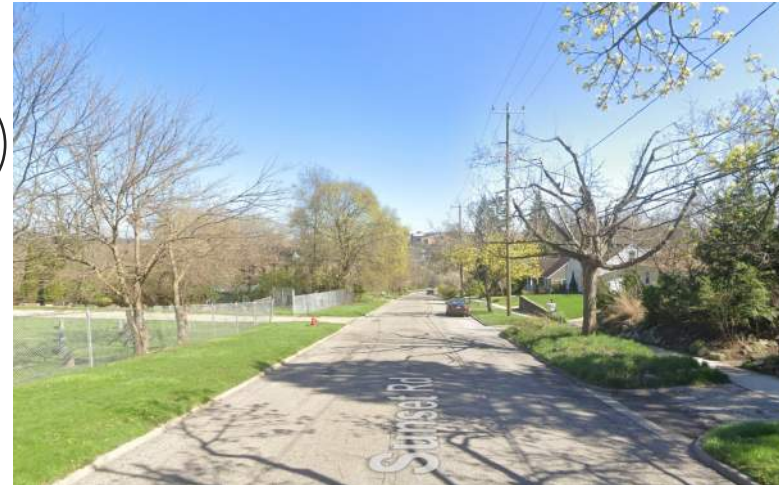
300 Sunset Rd - Existing Condition: North side of Sunset Rd, looking east
