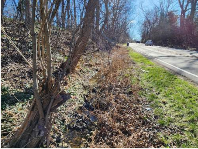
C1 Existing Condition: North side of Geddes Rd, looking east
