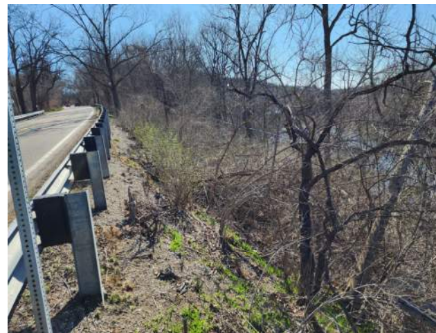
B2 Existing Condition: South side of Geddes Rd, looking east
