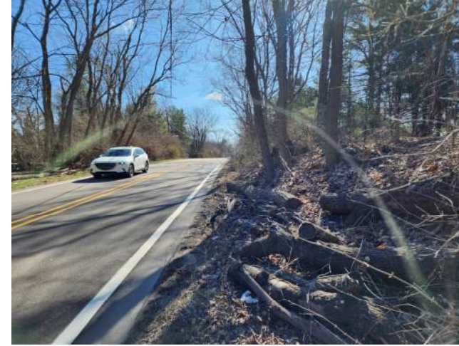
C2 Existing Condition: South side of Geddes Rd, looking east
