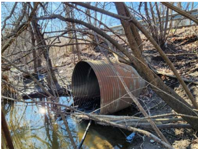
B1 Existing Condition: North side of Geddes Rd, looking east
