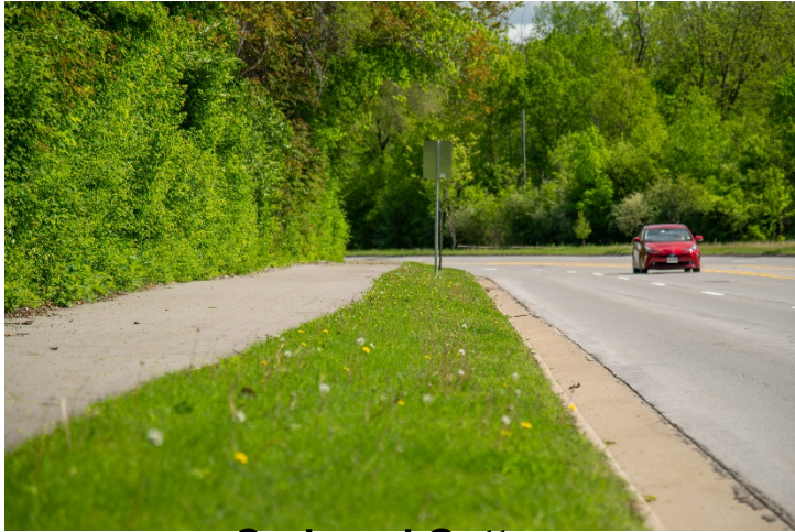
Curb and Gutter
