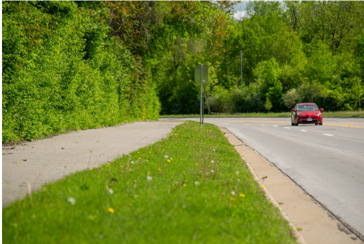
Curb and Gutter
